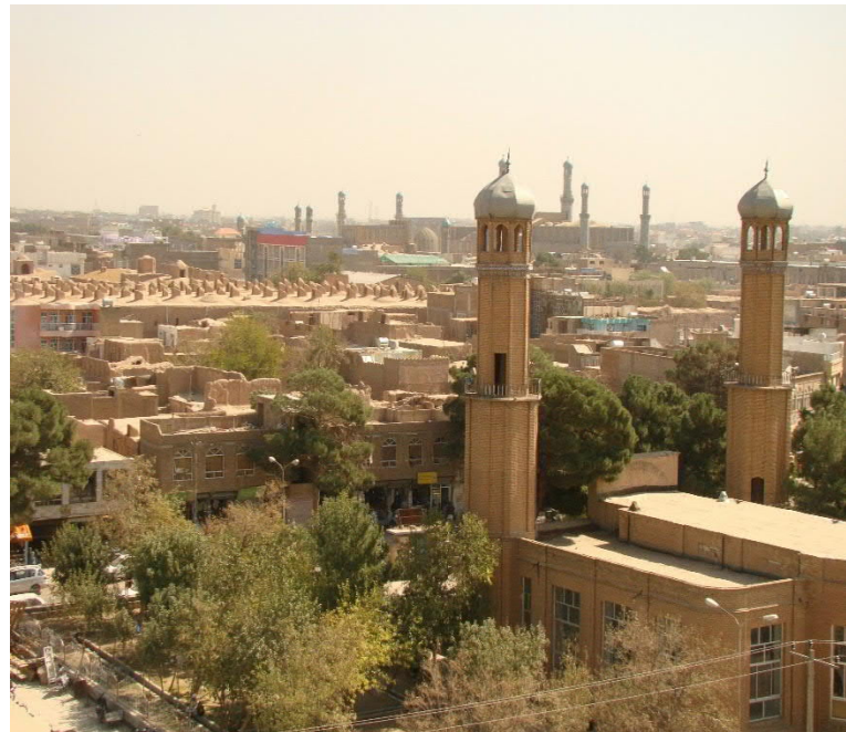
Fig. 3. Historic urban fabric of Herat. (© R. Sharifi)
