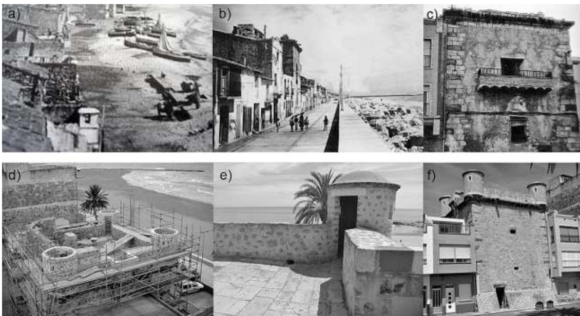
Fig. 3 – a), b), c), Fishing village, seafront limited (Copyright: www.todocoleccion.net) and front view, Torrenostra 's tower, sixteenth century. Copyright: (Boira, J.V., 2007). d), e) f),Restauration and current state, twentieth century (Copyright: Giraudeau, S. & Leonardi, A., 2015)
