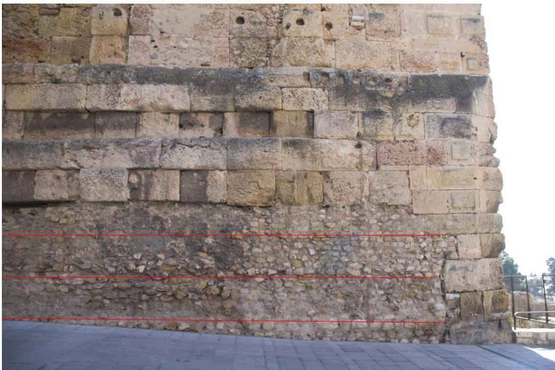
Fig. 10 – Part of the mixed foundations of the tower (Copyright: M. Serena Vinci)
