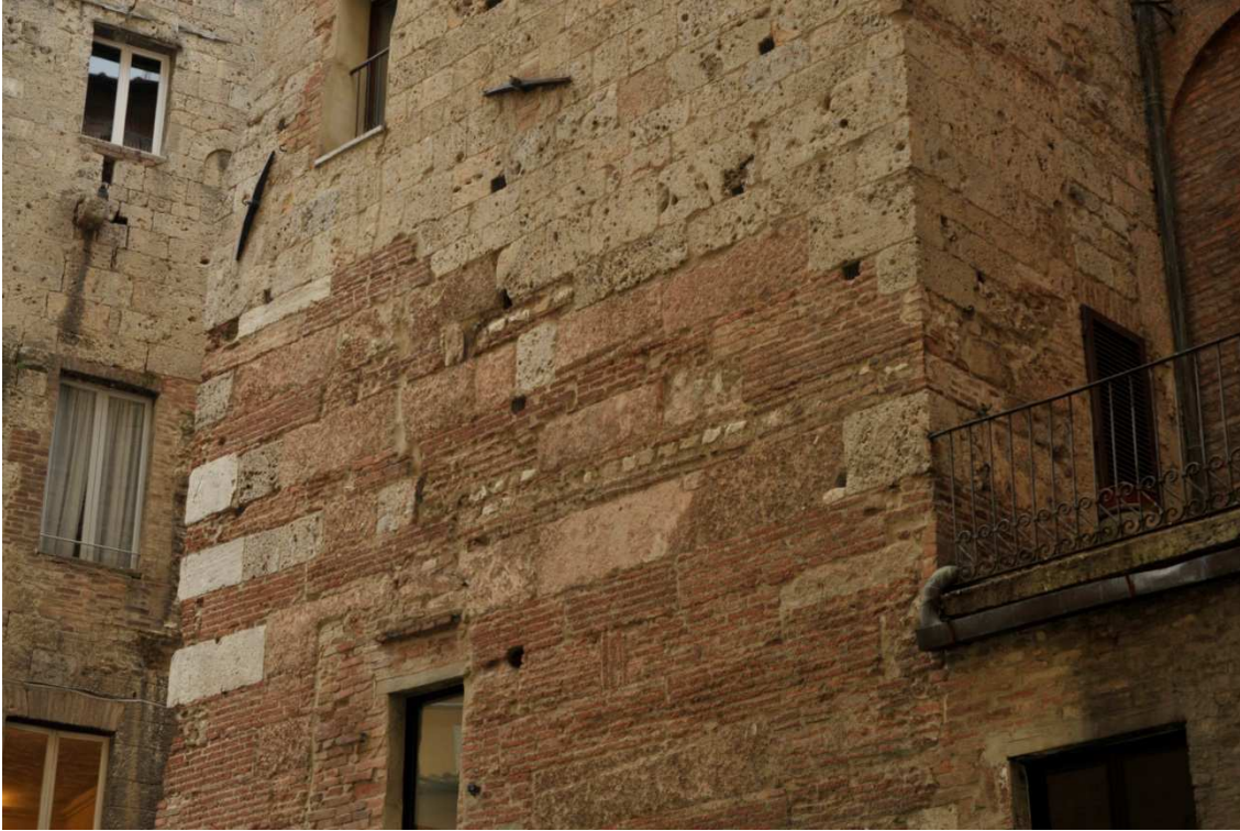
Fig. 8 – South wall of the east tower, built with reused materials.
