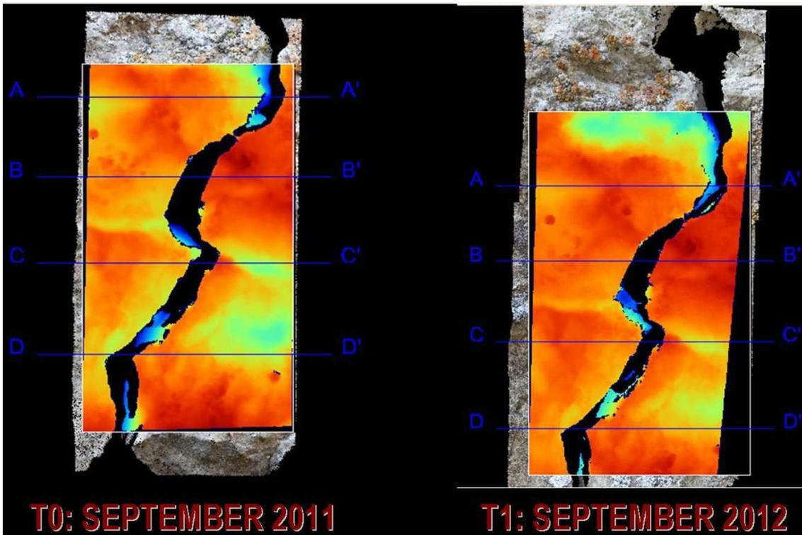
Fig. 7 – 3D models, DEM and sections of the crack in the church of Saint Gavino Adimari, all obtained through the ZScan Micro technology.
