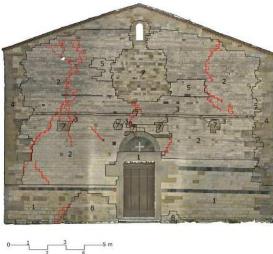
Fig. 4 – Example of orthophoto plan with a stratigraphic survey in phases (black lines) and crack framework (red lines) of the entrance façade of the Parish Church of Saint Agata in the Mugello. It is interesting that several damages run along the interfaces dividing different building phases. It is also interesting that some of these damages are concentrated only on some of the building phases rather than on others. This helped to date the phases and agencies found.
