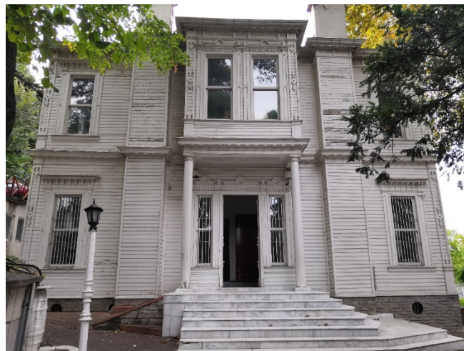
Fig. 1. Southeastern Façade of the Building and the Main Entrance, Bursa, Turkey (© Oğuz Yeke).
