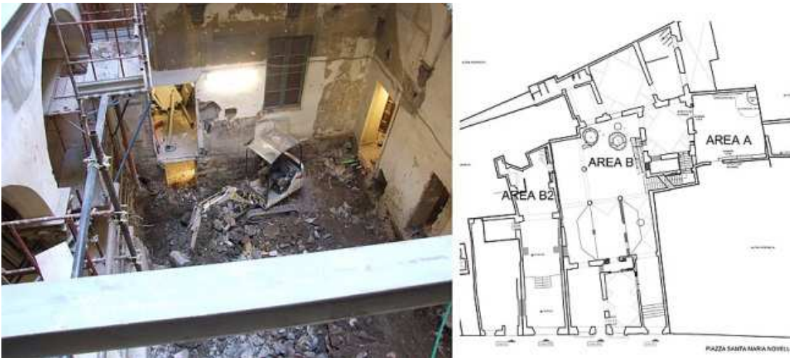
Fig. 2 – Plan of the ground floor with designated three areas of excavation. On the left picture of the area chosen
