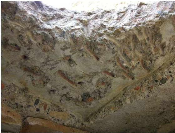
Fig. 9 – traces left by the lead nailed sheet
