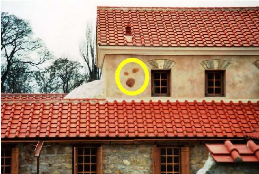
Fig. 10 – AP Carnuntum, condensate stains (sooting) at the easternmost side of the "Apsisraum" of the villa urbana © H. Lehar 2010
