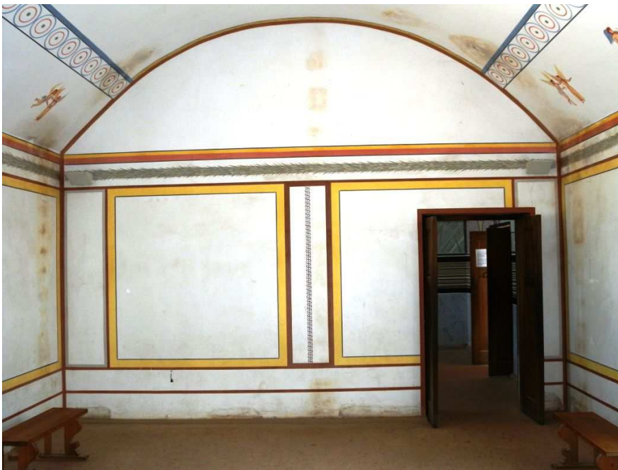
Fig. 11 – AP Xanten; walls of the tepidarium in the lodging house thermae show strong sooting. These stains make it easy to trace the route of the vents towards the vaulted ceiling © H. Lehar 2010
