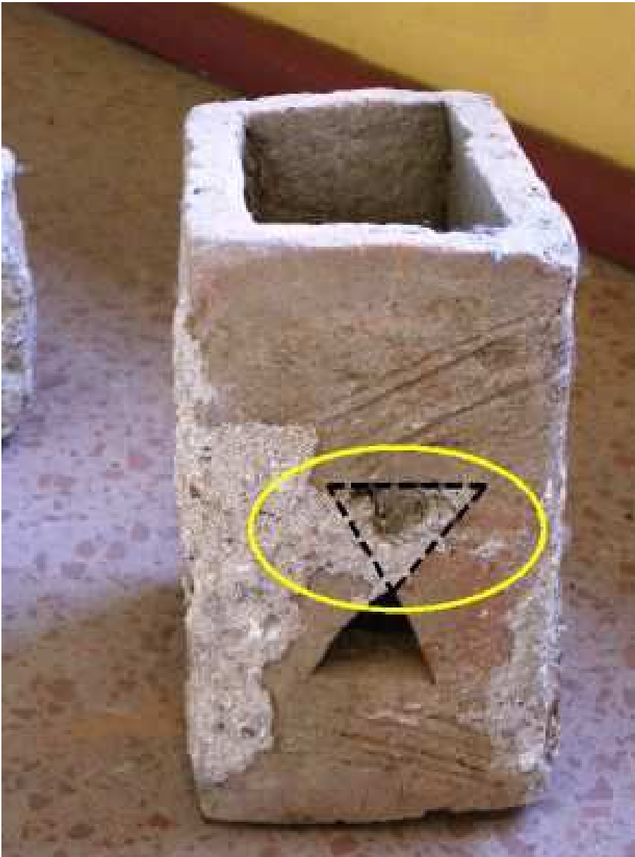
Fig. 6 – box flue tile with lateral openings. Remains of mortar show where it encroached the hourglass-shaped openings. This indicates possible use as a flue. AP Römische Villa Borg, museum © H. Lehar 2009
