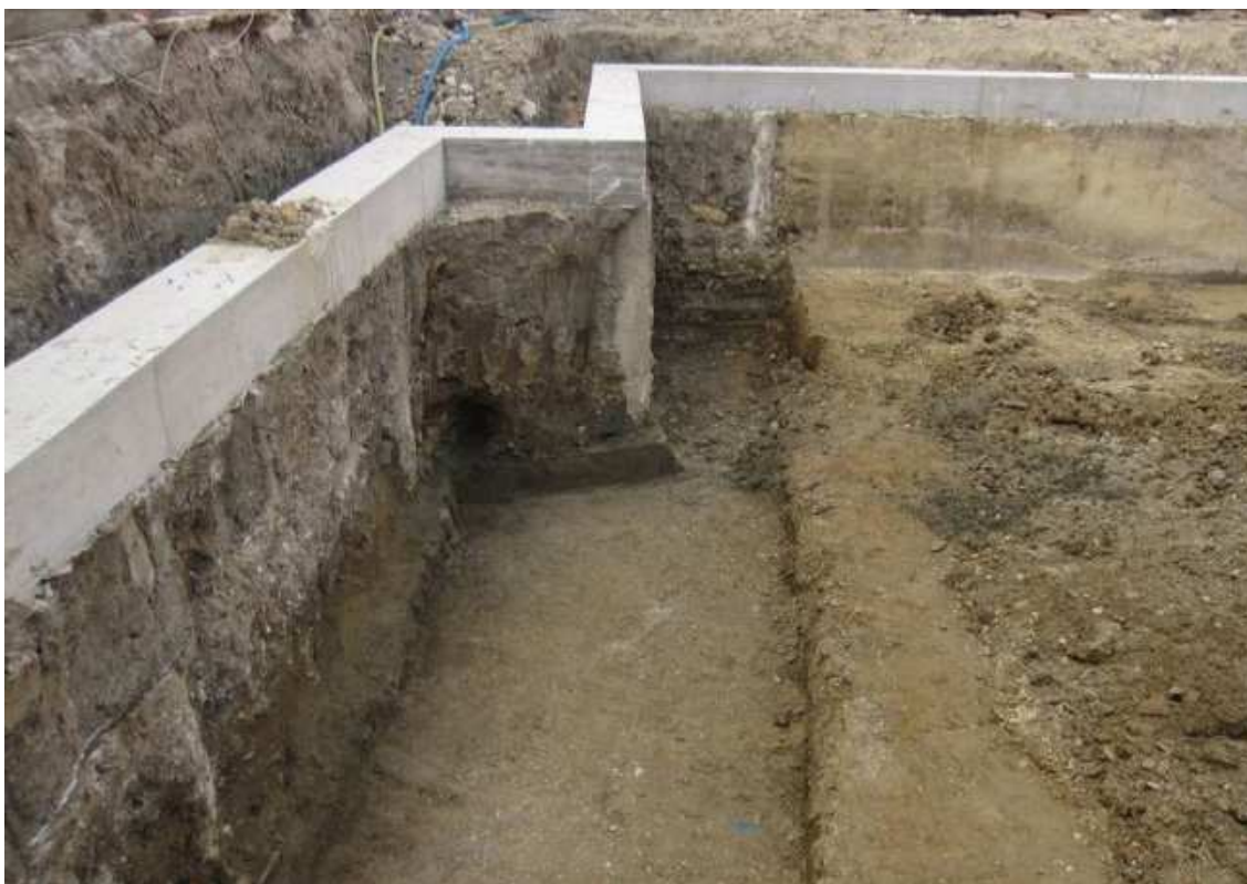
Fig. 7 – A detail of the northern section and of the trench for the foundation of the urban walls.
