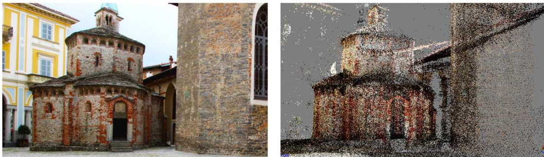
Fig. 5 – Baptistery of Biella – picture and point cloud (Copyright: Angela Mancuso, Andrea Pasquali)
