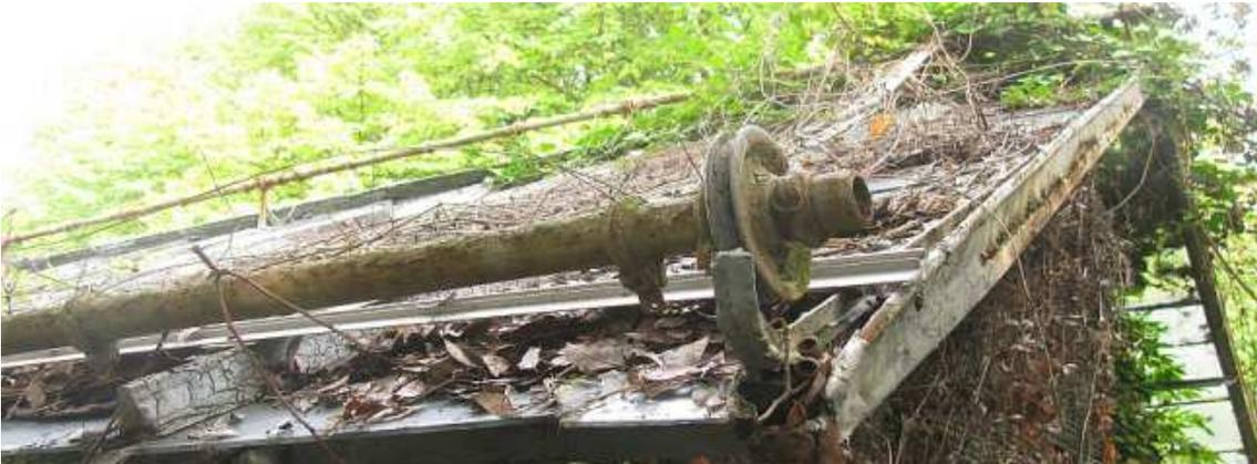
Fig. 9 – Pulley system, Serre La Torretta, Montecatini (Copyright: Valentina Fantini)
